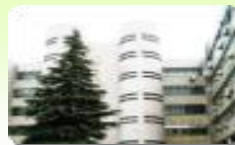
APLEX China branch Shanghai, China
